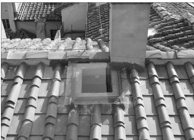
Fig. 9. The skylight set into the roof.
